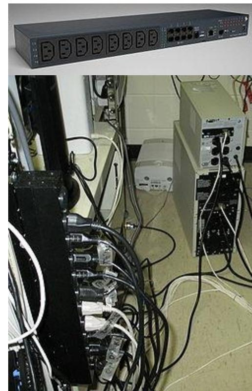
A 10-outlet rack-mount PDU without built-in surge protection, connected to a UPS (bottom unit on right)
