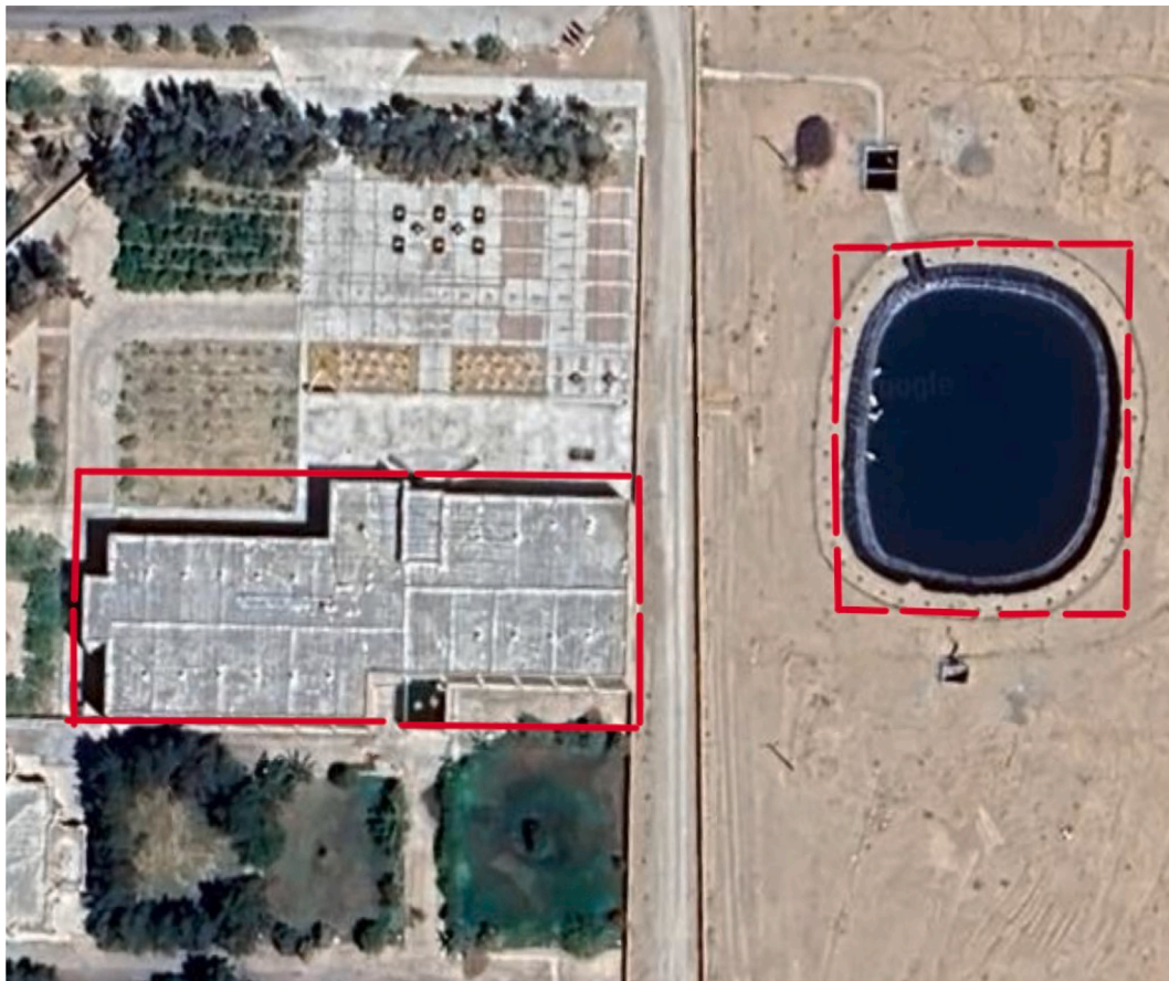
Fig. 3. The location of the solar power plant in the IAUN Science and Technology Park campus building using the Google Earth map [13].
